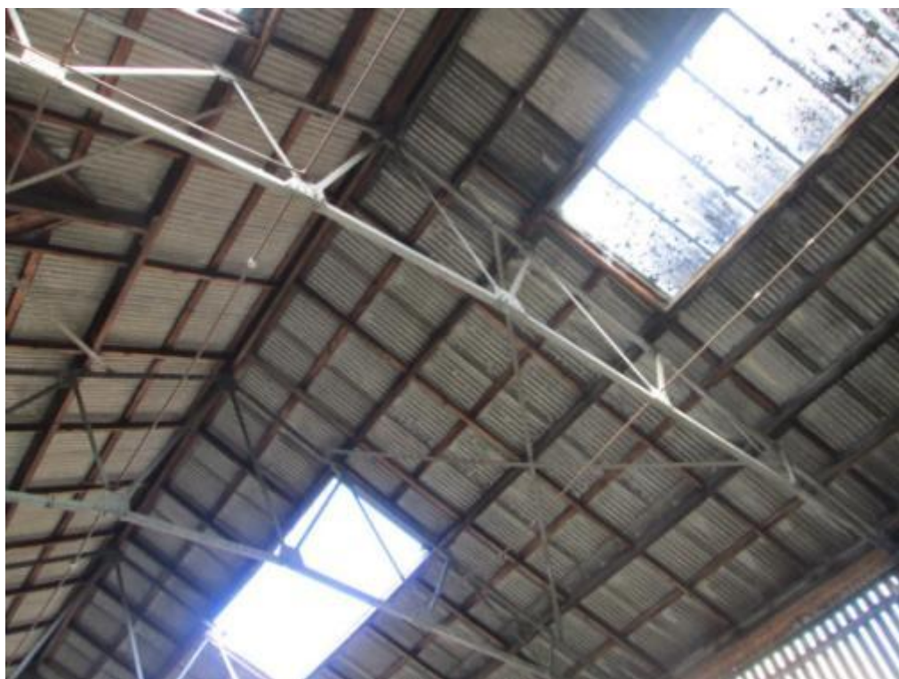
Photograph 53 – Cross bracing in roof
