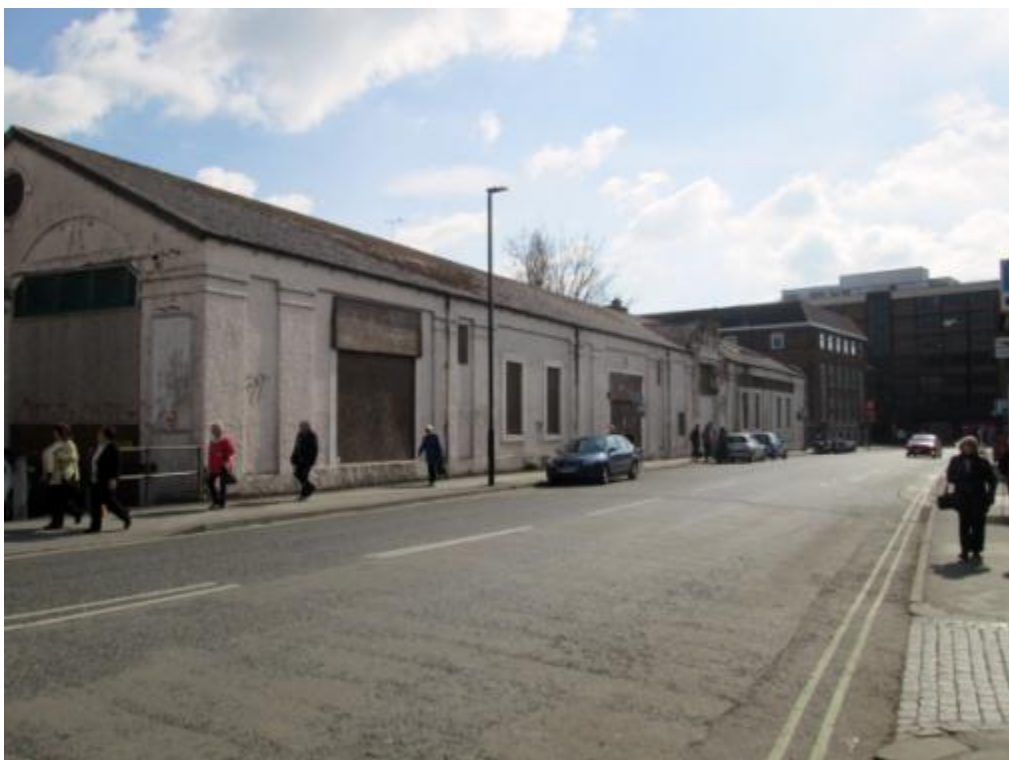
Photograph No. 2 – Piccadilly elevation
