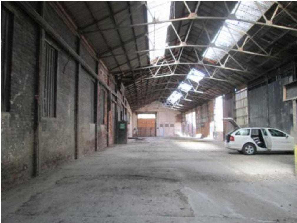
Photograph 61 – Internal view from Dennis Street
