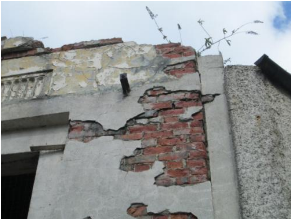
Photograph No. 31a – Part Dennis Street entrance elevation
