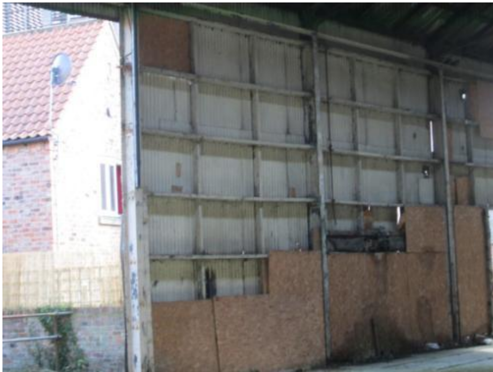
Photograph 40 – Part view on rear elevation
