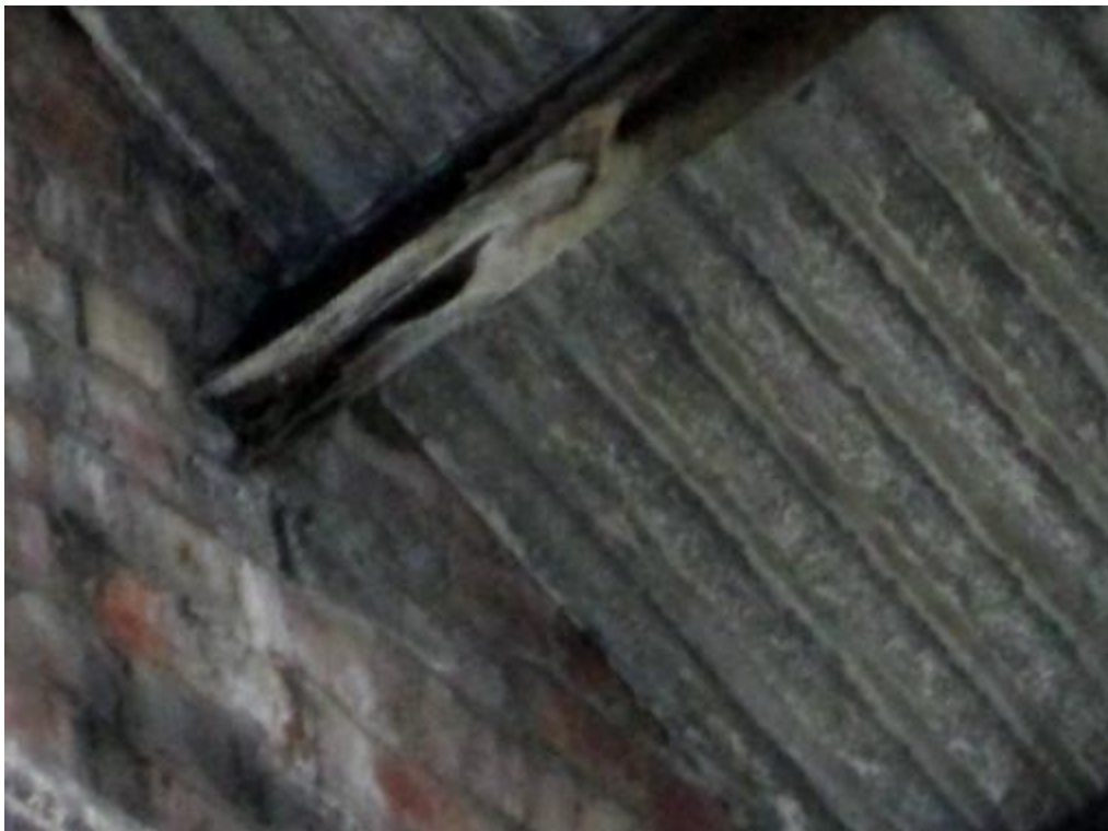
Photograph 47 – Purlin bearing into wall above Piccadilly entrance
