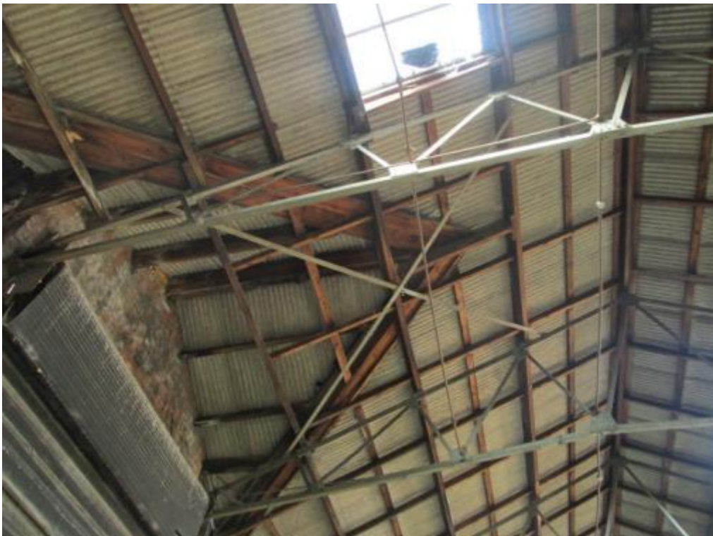
Photograph 52 – Cross bracing in roof
