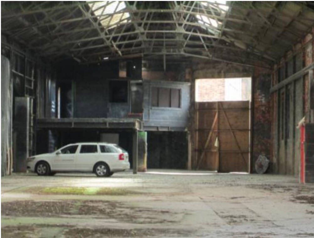
Photograph 59 – Internal view towards Denis Street
