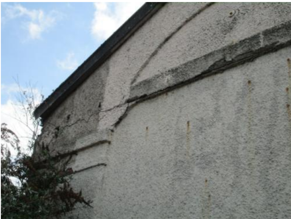
Photograph No. 28 – Part North West elevation
