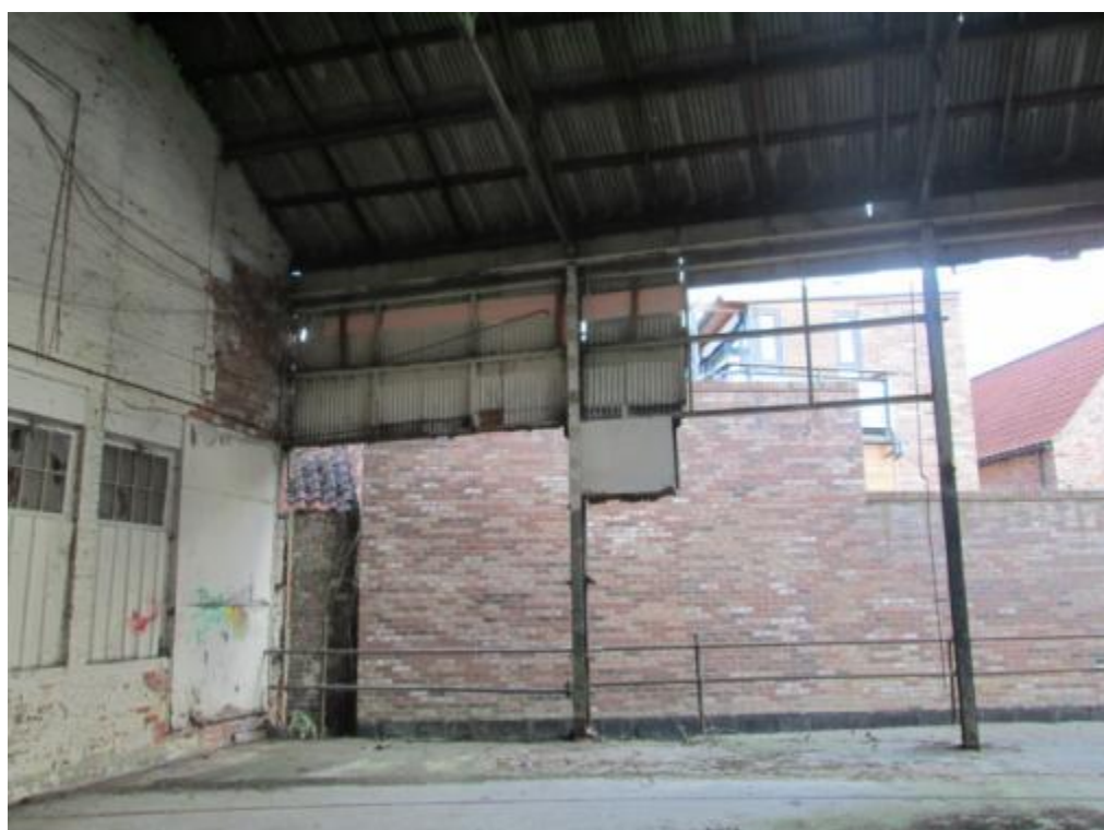
Photograph 39 – Part view on rear elevation
