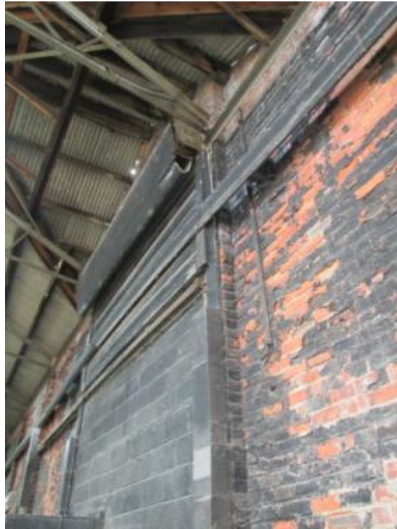
Photograph 36a – Internal view above Piccadilly entrance
