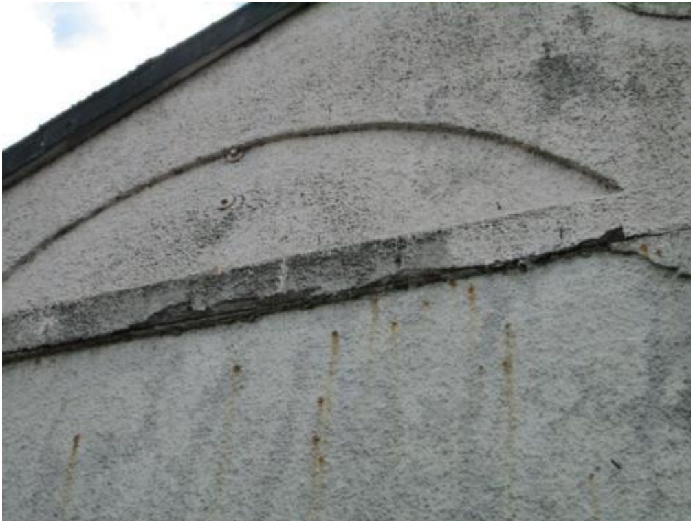
Photograph No. 27– Part North West elevation
