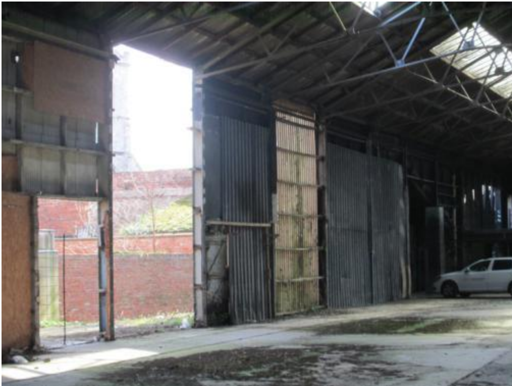
Photograph 41a – Part view on rear elevation
