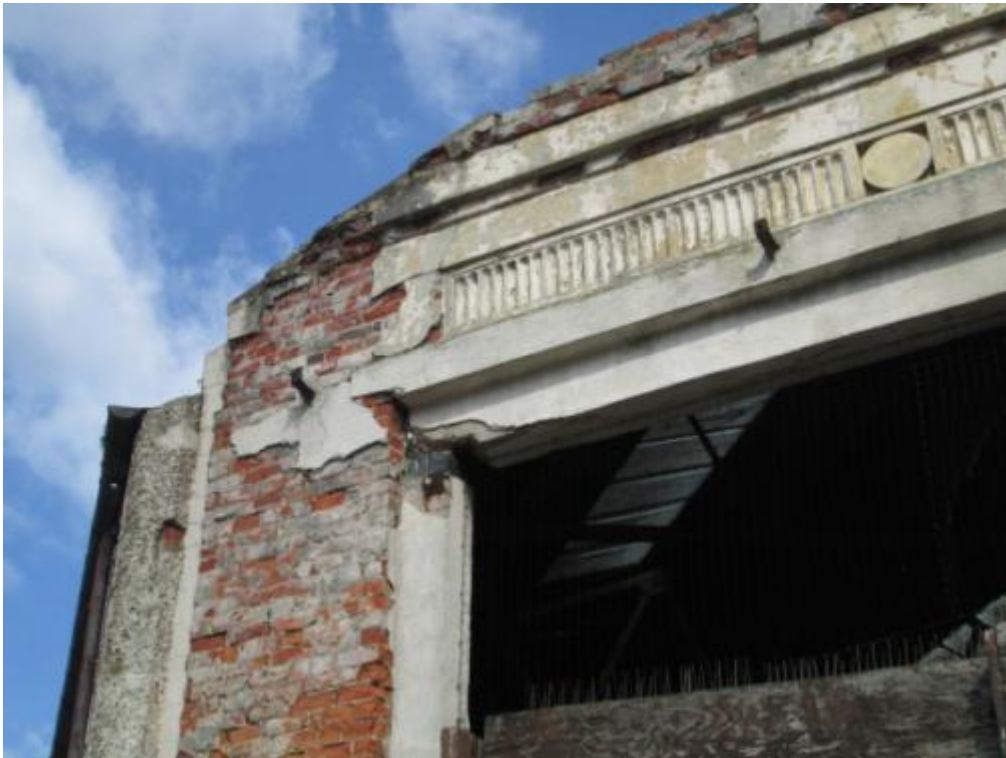
Photograph No. 31 – Part Dennis Street entrance elevation
