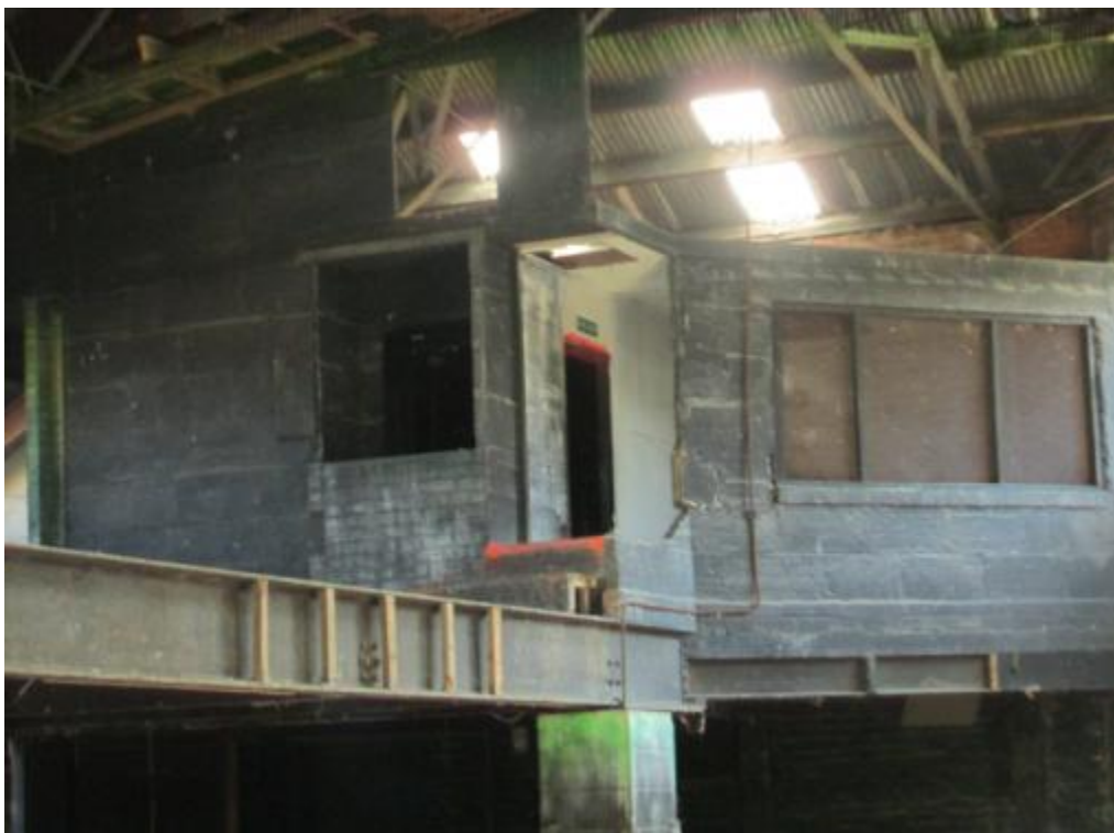
Photograph 42 – Partially demolished wall at Dennis Street
