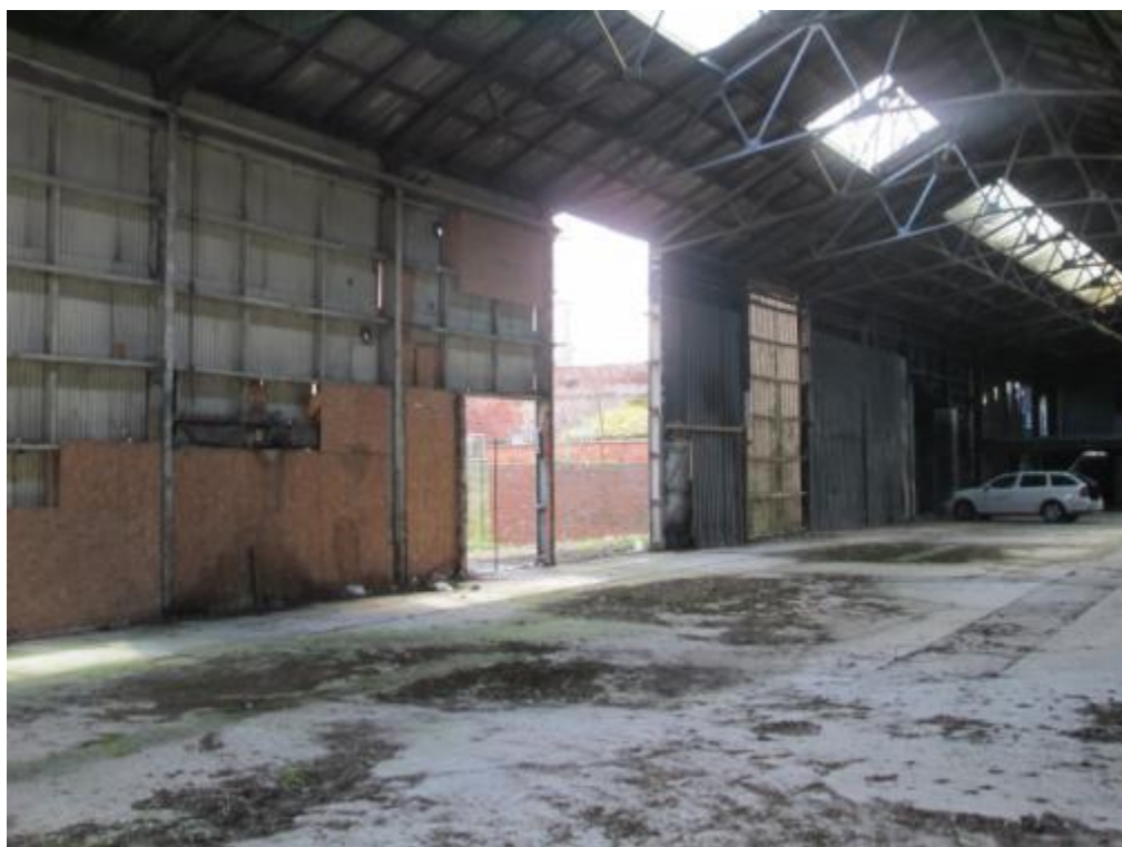
Photograph 41 – Part view on rear elevation
