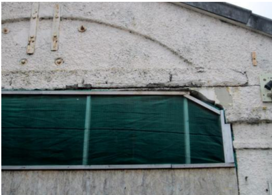
Photograph No. 24 – Part North West elevation
