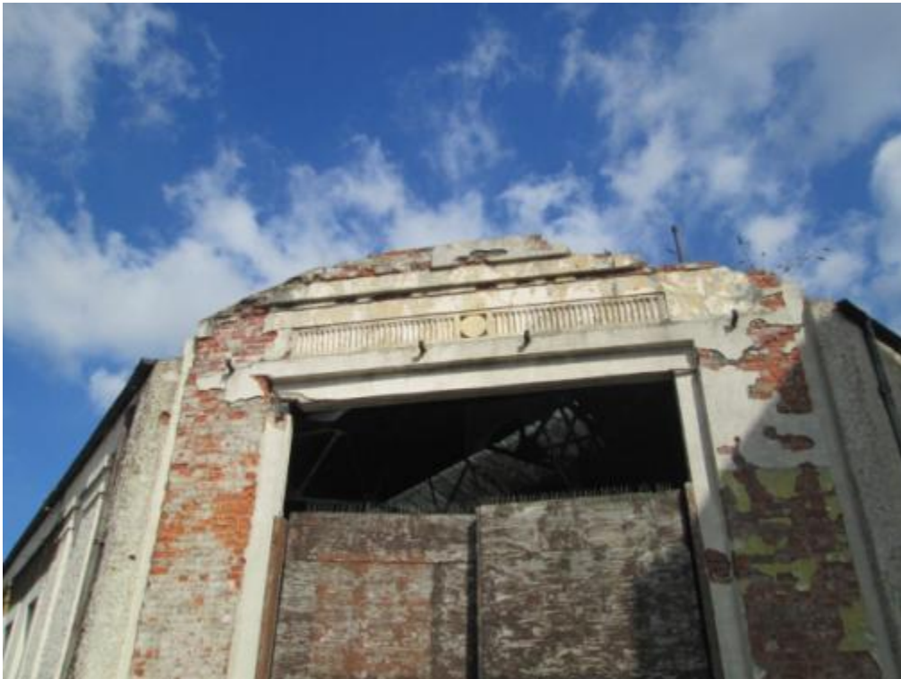
Photograph No. 30 – Dennis Street entrance elevation
