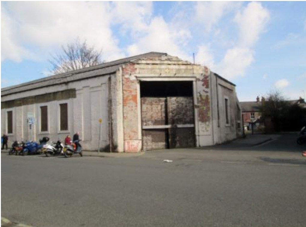
Photograph No. 3 – Dennis Street elevation
