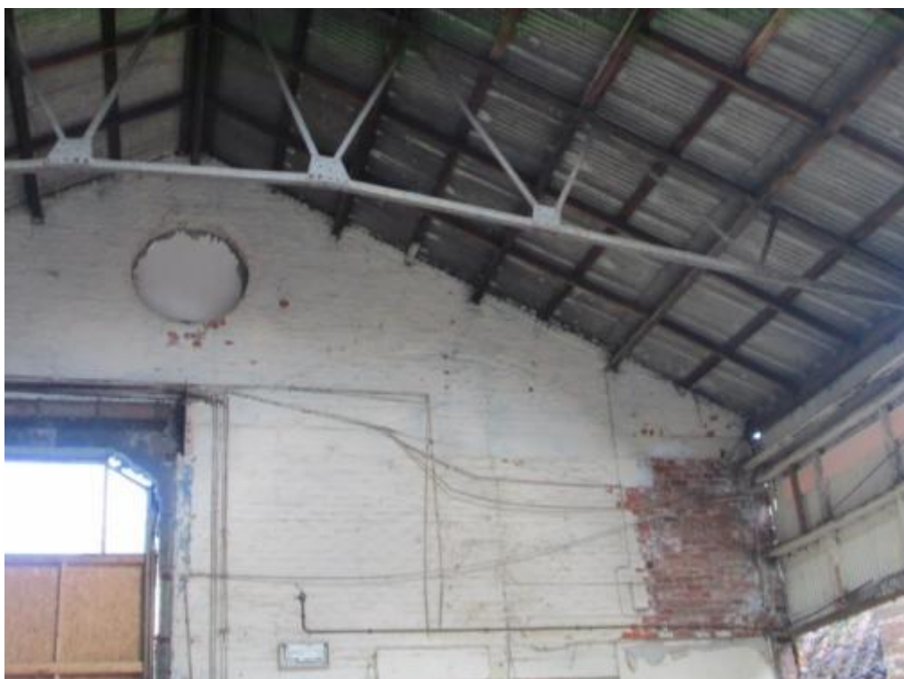
Photograph 38 – Internal view towards North West entrance
