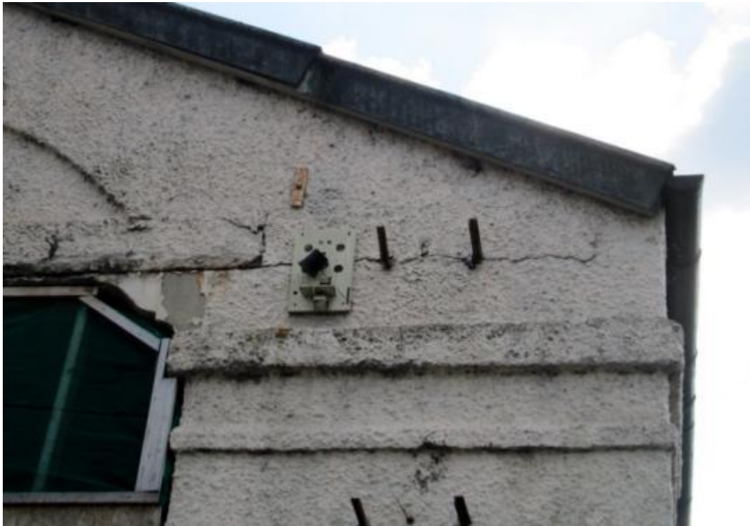
Photograph No. 23 – Part North West elevation
