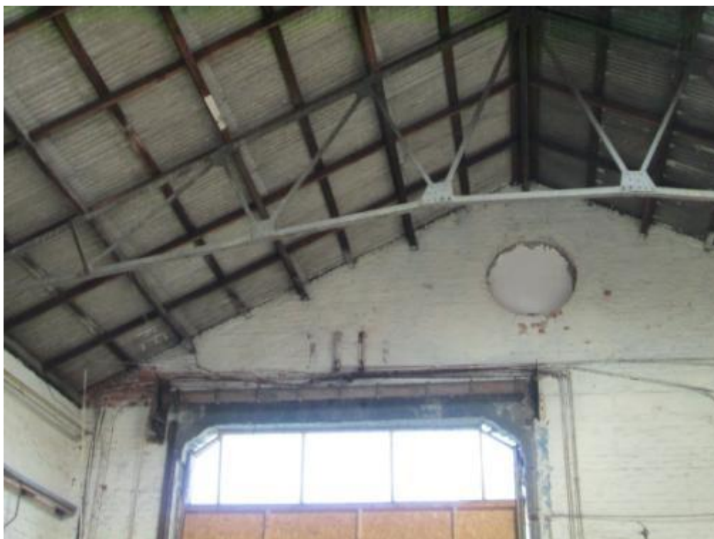
Photograph 37 – Internal view towards North West entrance
