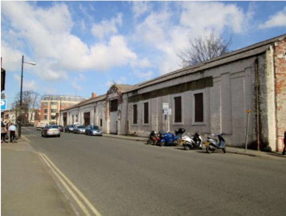
Photograph No. 1 – Piccadilly elevation
