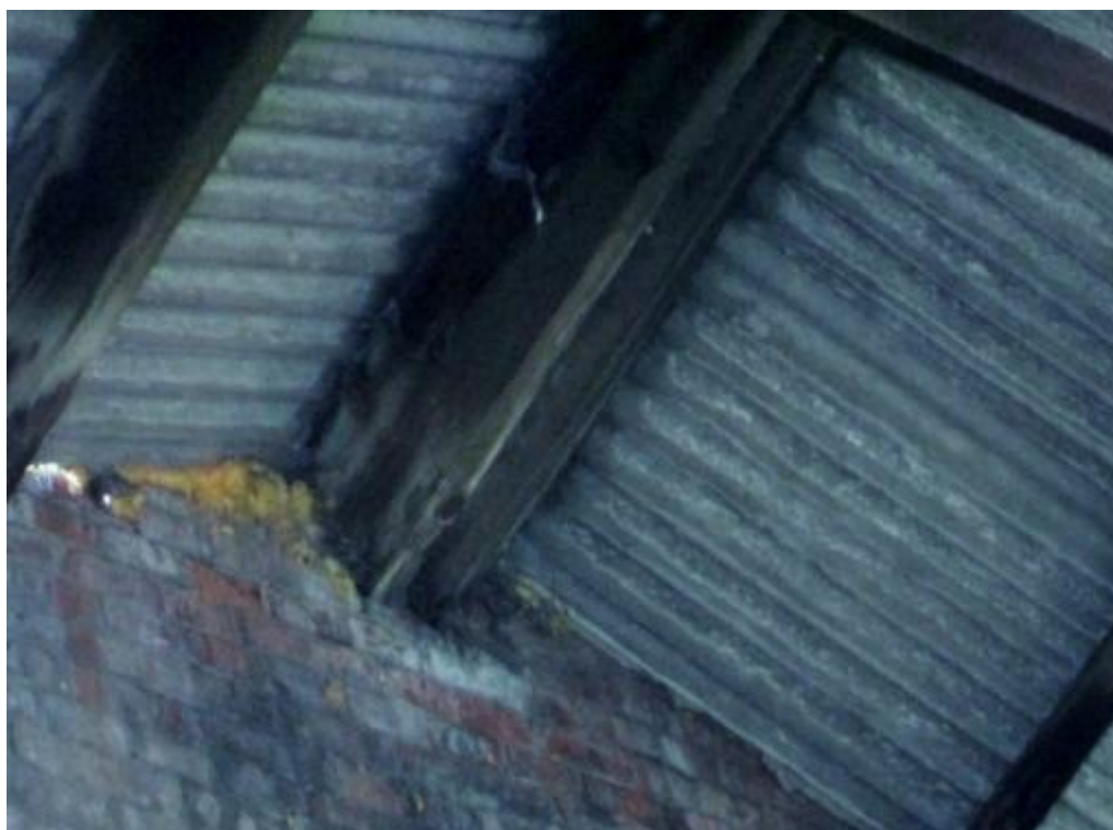
Photograph 49 – Purlins bearing into wall above Piccadilly entrance
