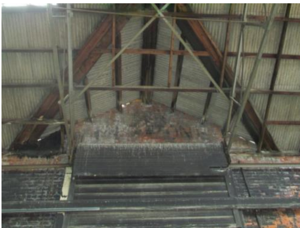
Photograph No. 36 – Internal view above Piccadilly entrance
