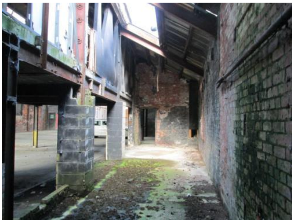
Photograph 62 – Internal view within lean-to looking from Dennis Street end
